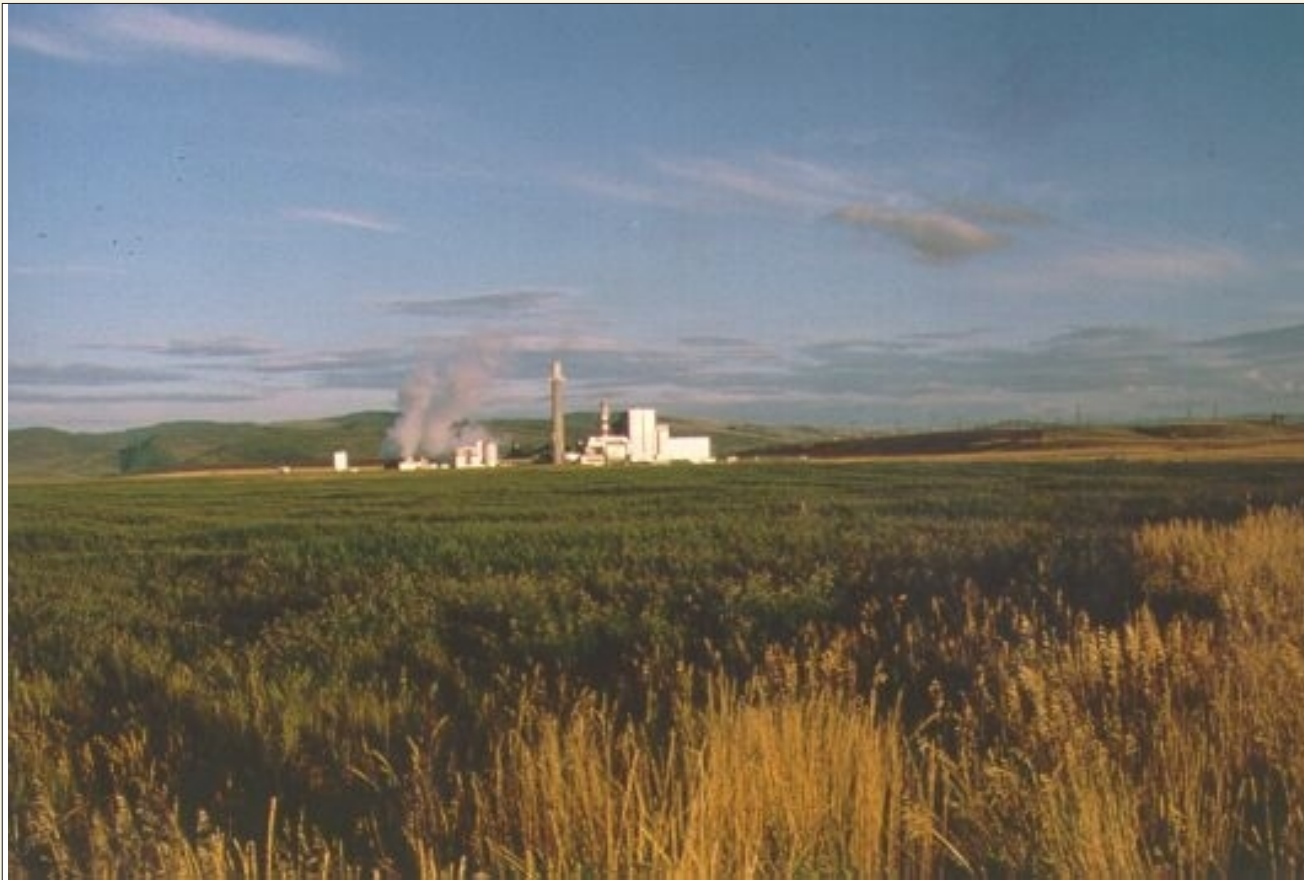
Hayden Power Plant
